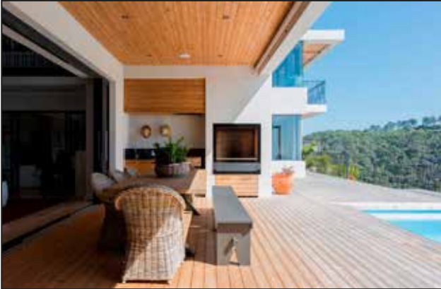
The year of construction 2020, South Africa. The graying process has begun. The boards most exposed to UV radiation start first to fade. Part of them very uneven. This is due to the inherent properties of wood and their variation.
