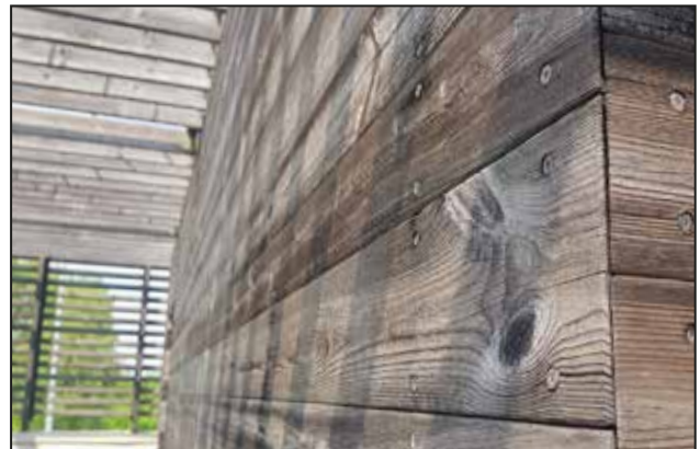
The year of construction 2009, photo 2019, Italy. Although the graying process has reached its end point, there are still shade variations in the surface according to the variation in the natural properties of the wood.
