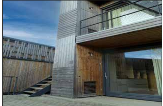
The year of construction 2020, photo 2022, the Netherlands. The compass point also affects the progress of the graying process. The color can sometimes be partially or completely black. Momentary humidity conditions also affect the prevailing tone of shades. The installation direction also affects the speed of the process.
