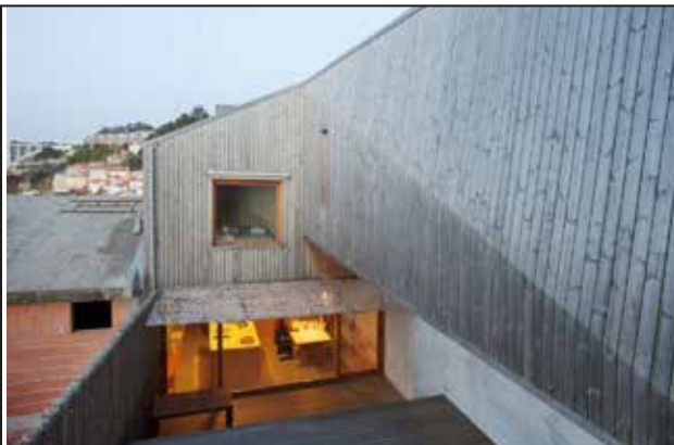
The year of construction 2015, photo 2019, Portugal. The surface has taken on a beautiful silver-gray hue. The part of the wall in the shady area has still retained its original, albeit faded tone.
